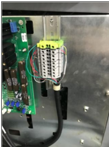
Fig.1.3 Relays Inside the CNC Controller
